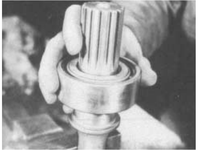
3. Fit the bearing on to the shaft with the radius of the inner bearing ring to the shaft collar.
