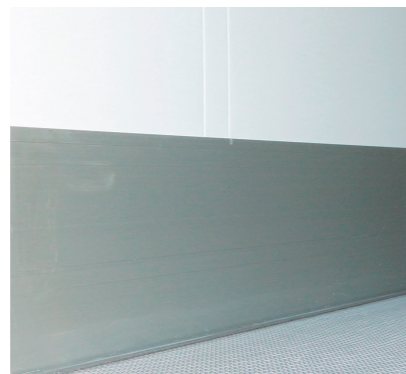
The fully welded all-around kick strip protects the floor from water ingress.
